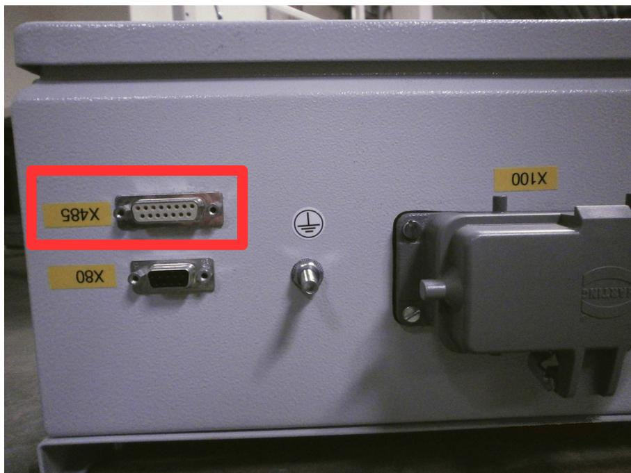
A removed or non working RS485-Bus will result in a communication error at IFP. If communication is lost for over 10 minutes the chiller will proceed with daymode.
