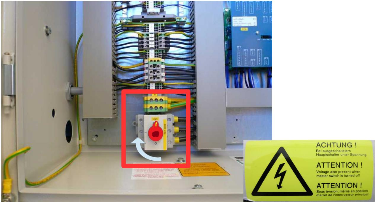
The power supply for the IFP is performed from MRI → connector X100.
