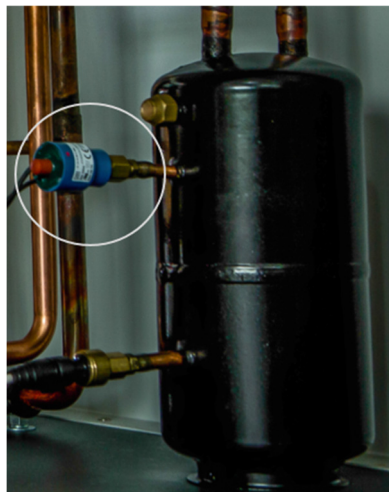
Figure 3 High Pressure Limiter Location
