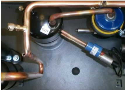
Figure 7: Position of the high-pressure limiter (PZH)
