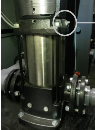
Figure 17: Position of the pump vent (vertical type)
