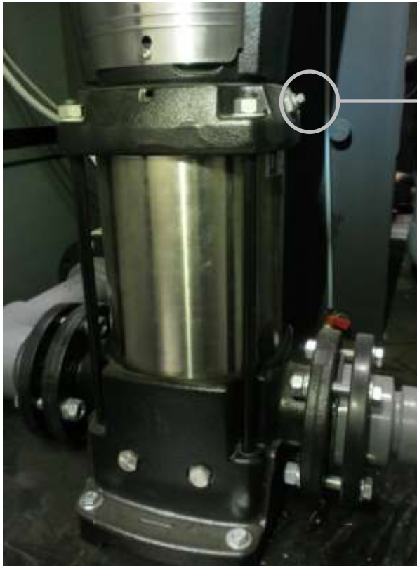
Figure 17: Position of the pump vent (vertical type)
